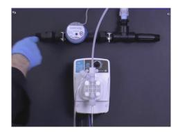
**Step 8:** Do this by running fresh water through the supply line and watching the dial for movement.
