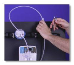
**Step 7:** Cut the rigid polyethylene discharge tubing so that it runs comfortably from the discharge valve to the injection valve. Set the remaining tubing aside.
