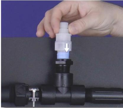
**Step 32:** Install and hand tighten the Injection Valve into the installation saddle or tee in the supply line. Do not overtighten.
