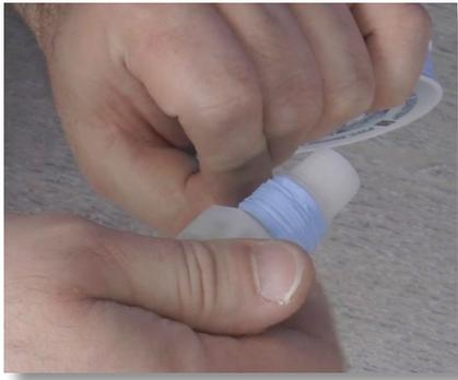
**Step 31:** Take the thread seal tape and wrap it around the threads of the Injection Valve for the necessary size – 3/8" or 1/2".
