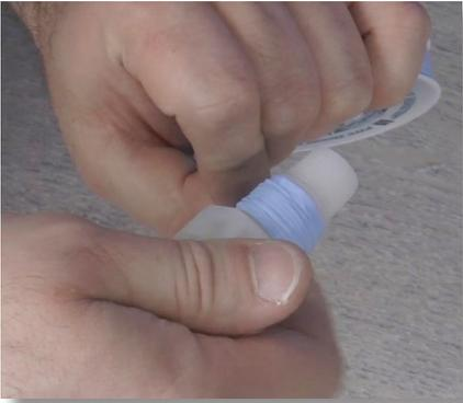
**Step 31:** Take the thread seal tape and wrap it around the threads of the Injection Valve for the necessary size – 3/8" or 1/2".
